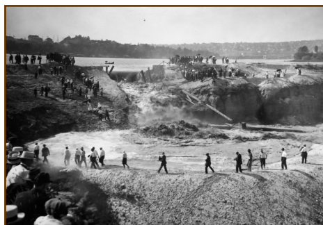
Workers completing the last part of the Lake Washington Ship Canal (looking southeast)
