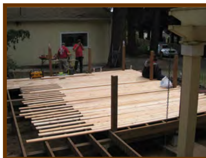
The deck is ¾ done.
