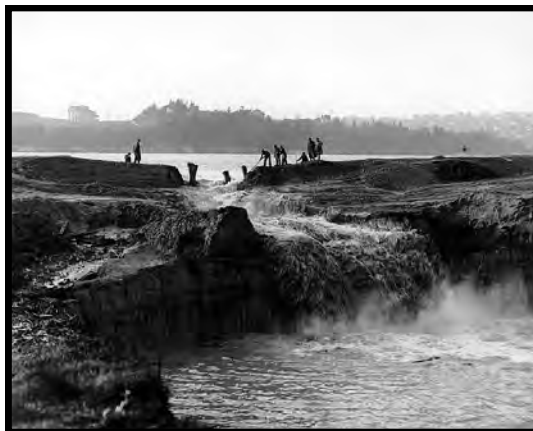
Cutting the coffer dam to let Lake Union into Lake Washington, December, 1913 University of Washington Special Collections
