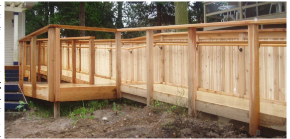
The completed ADA ramp will allow our guest with special needs easier access to the DeYoung House and Museum.
