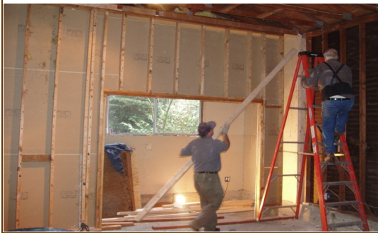
Earl Gray hands a supporting stud to Jim Kraft (on the ladder) after this portion of the back wall in the garage had been moved three feet.
