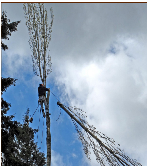
Removal of the poplar tree makes way for a new sidewalk at the DeYoung House.
