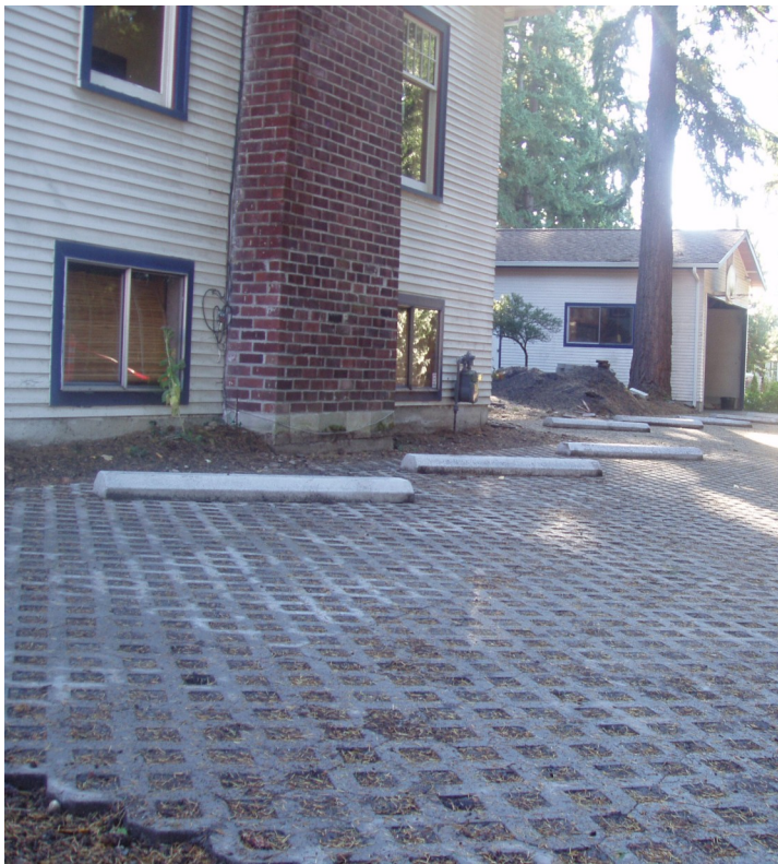
A few of the ten new parking spaces at the DeYoung House with semi-permeable pavers to allow water drainage. This photo has been made possible by Jim Kraft.
